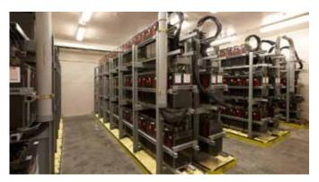
Wet-cell batteries in a large battery room application.
