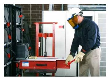
Appropriate personal protective equipment is essential when working on batteries or any UPS equipment.
